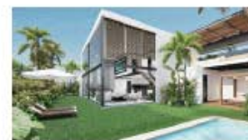
FACHADA POSTERIOR/BACK FACADE
